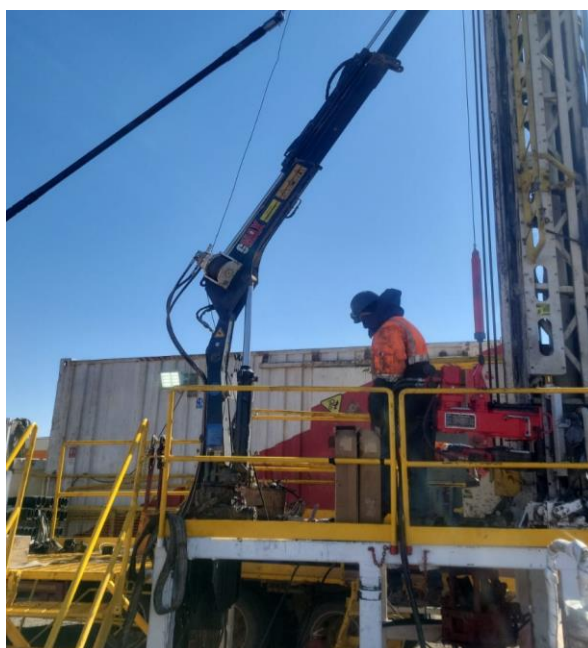
Workover rig at Nomgon-10
