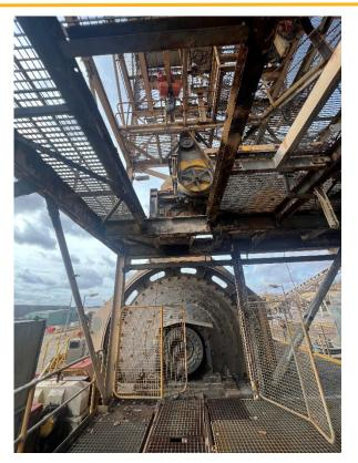
Figure 6 – Mill feed chute removed for rubber lining
