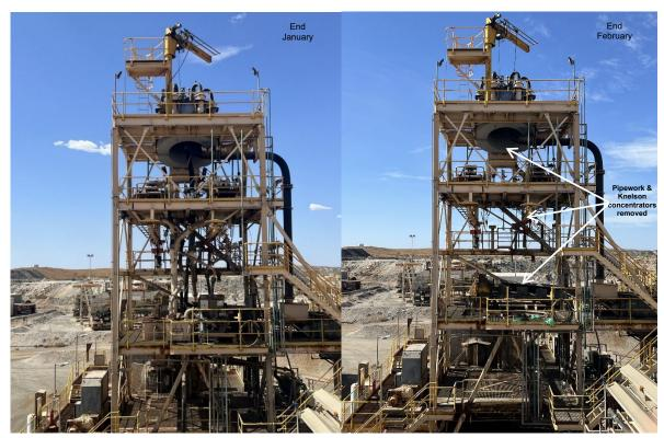
Figure 5 – Knelson concentrators along with cyclone underflow and mill feed pipework removed. Pipework will be rubber lined.
