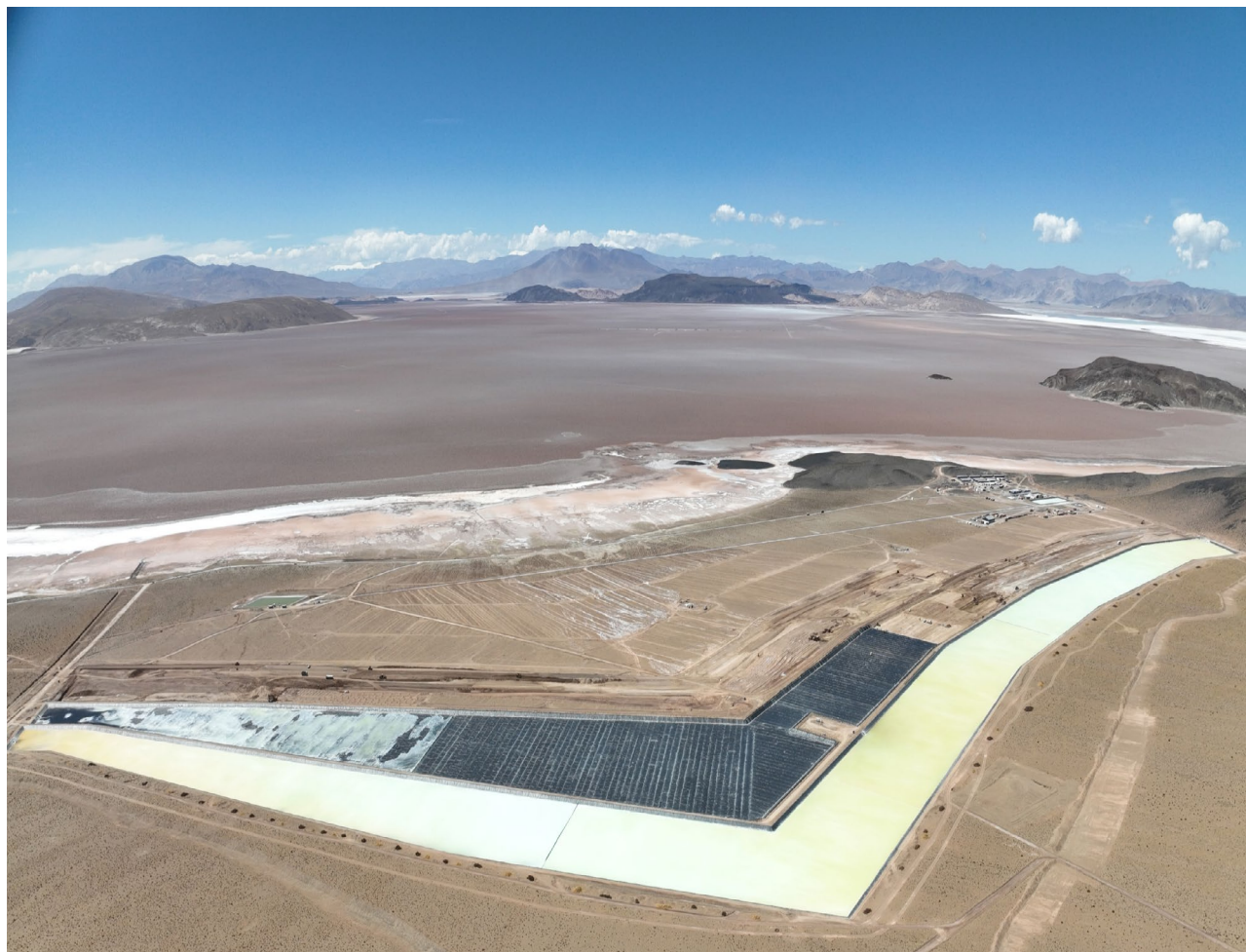
Pond 2 filling has commenced
