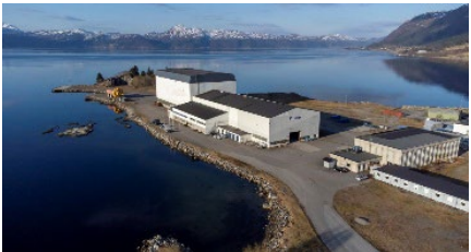
Prodtex Facility Fiska, Norway
