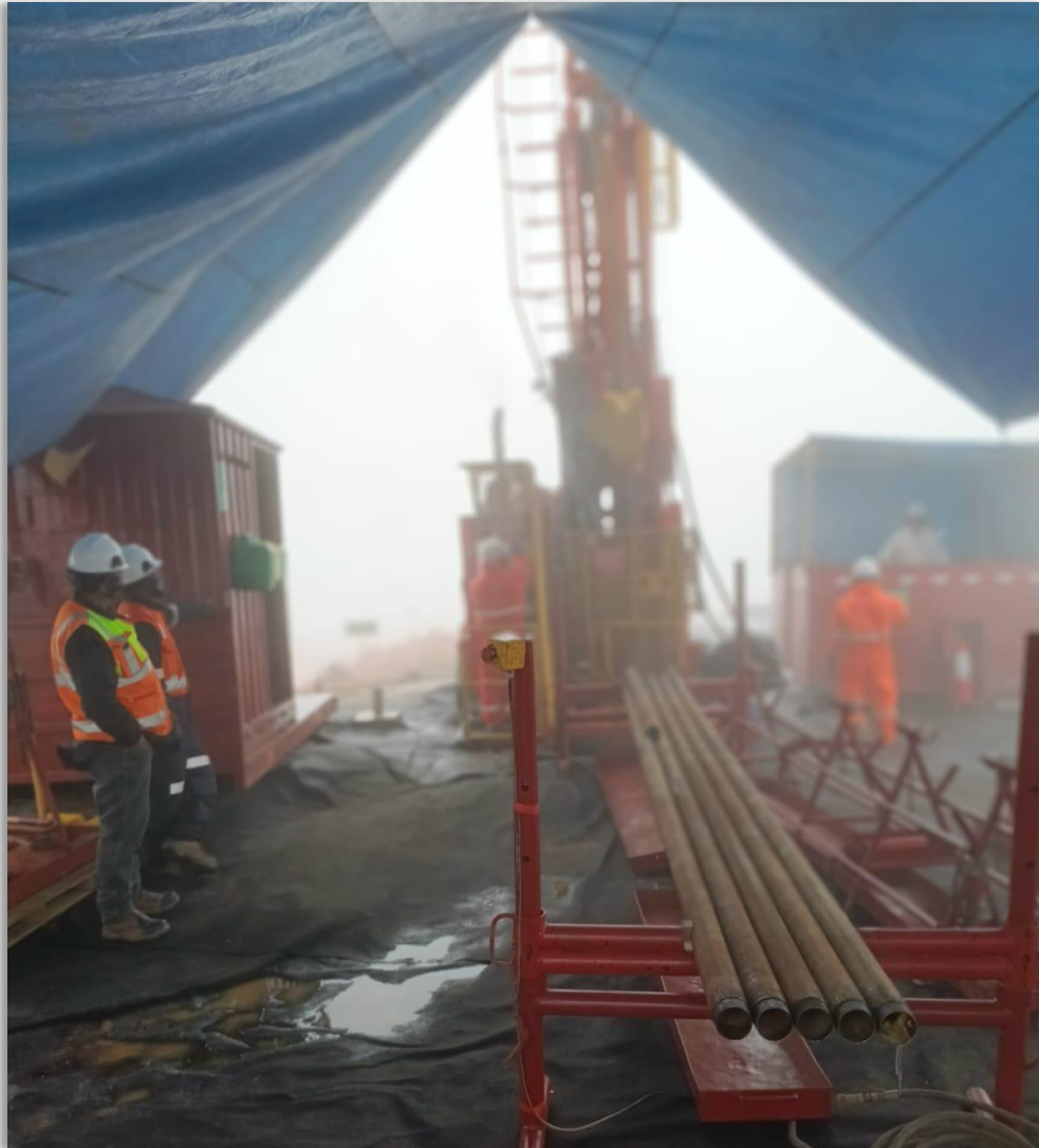
Figure 5. Drill Rig at Parag 25 th January 2024
