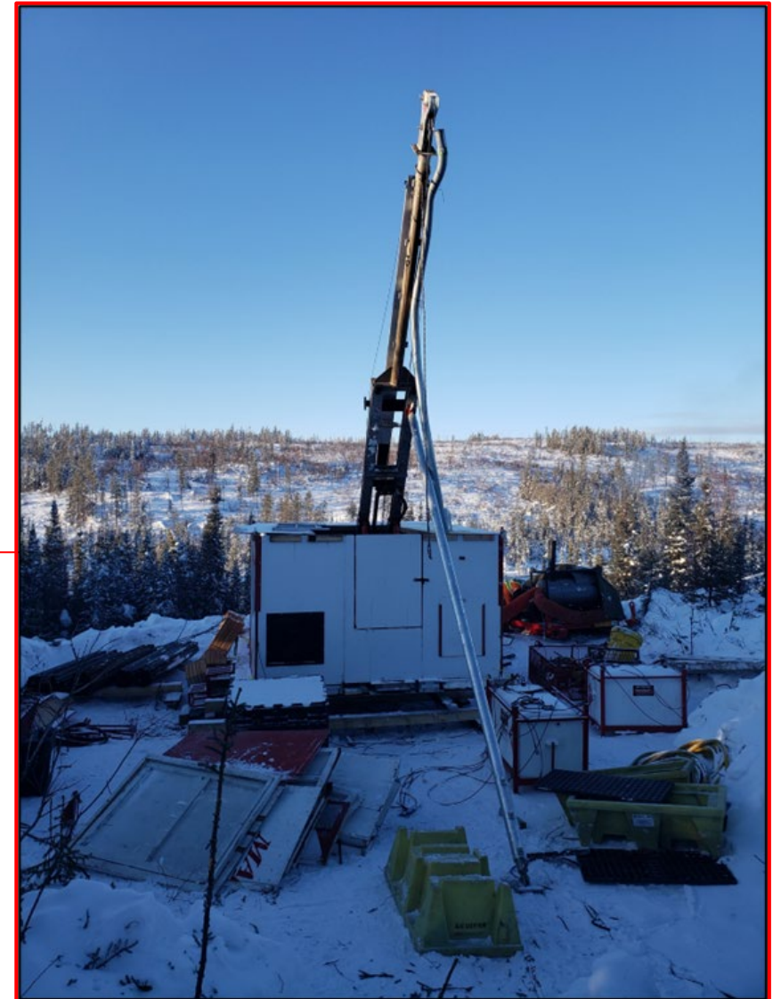
Drilling at Hook Lake Project
