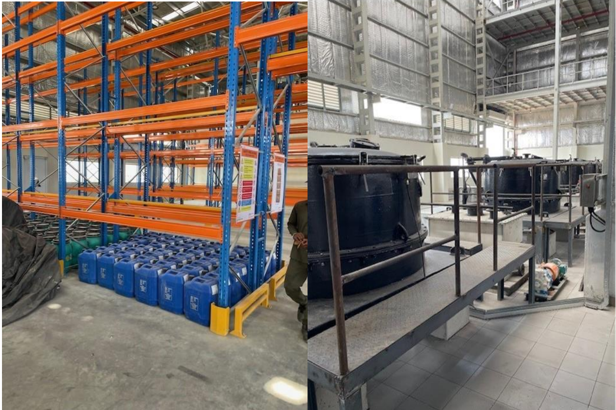
Figure 4 – various consumables and storage in place to accommodate over 1,000 tonne of material
