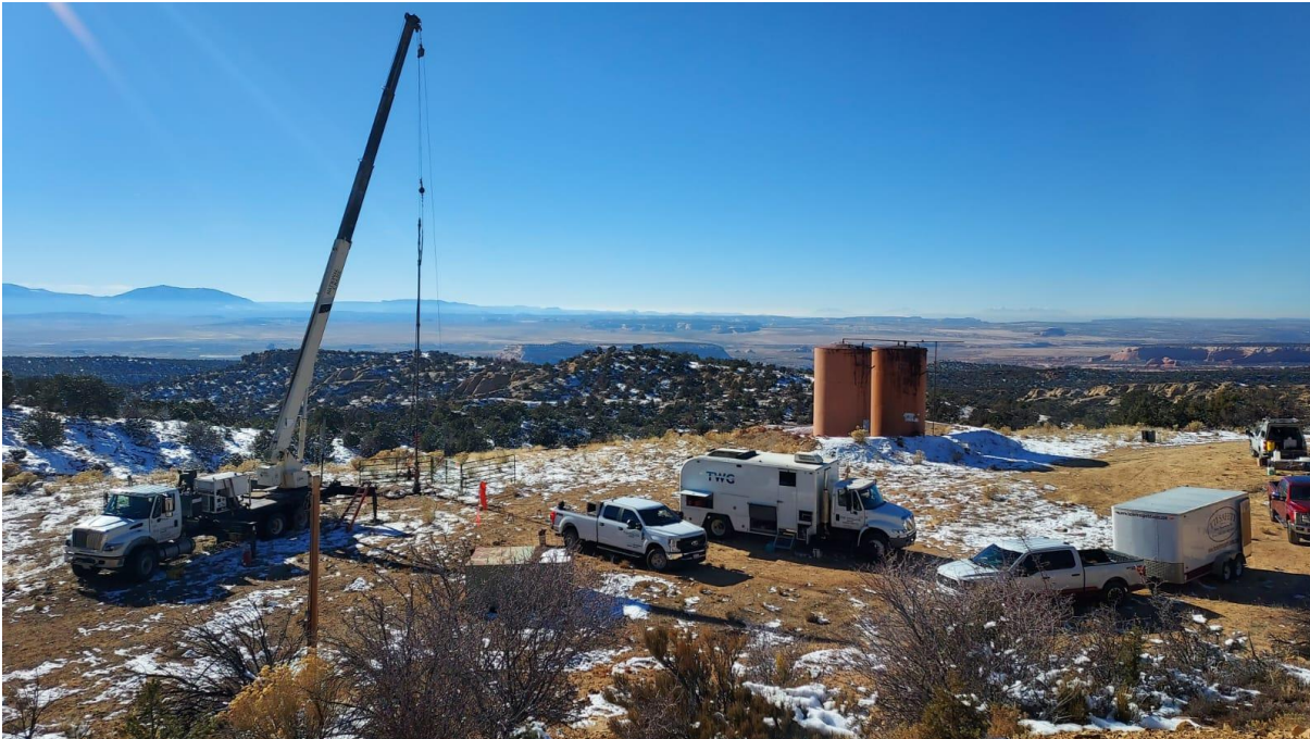
Figure 1. Wireline unit conducting brine sampling operations
