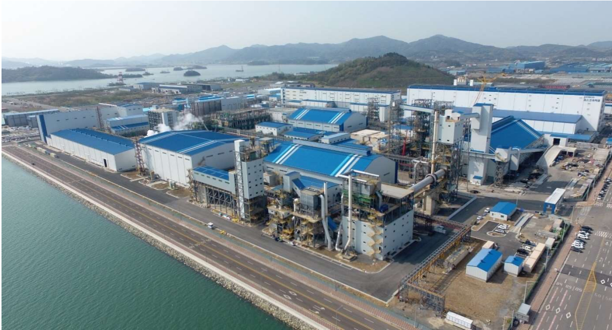
Figure 1: The PPLS LHM facility as at 12 April 2024.
