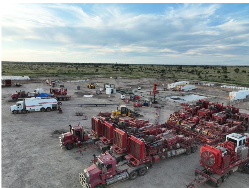
Halliburton fleet arriving on site
