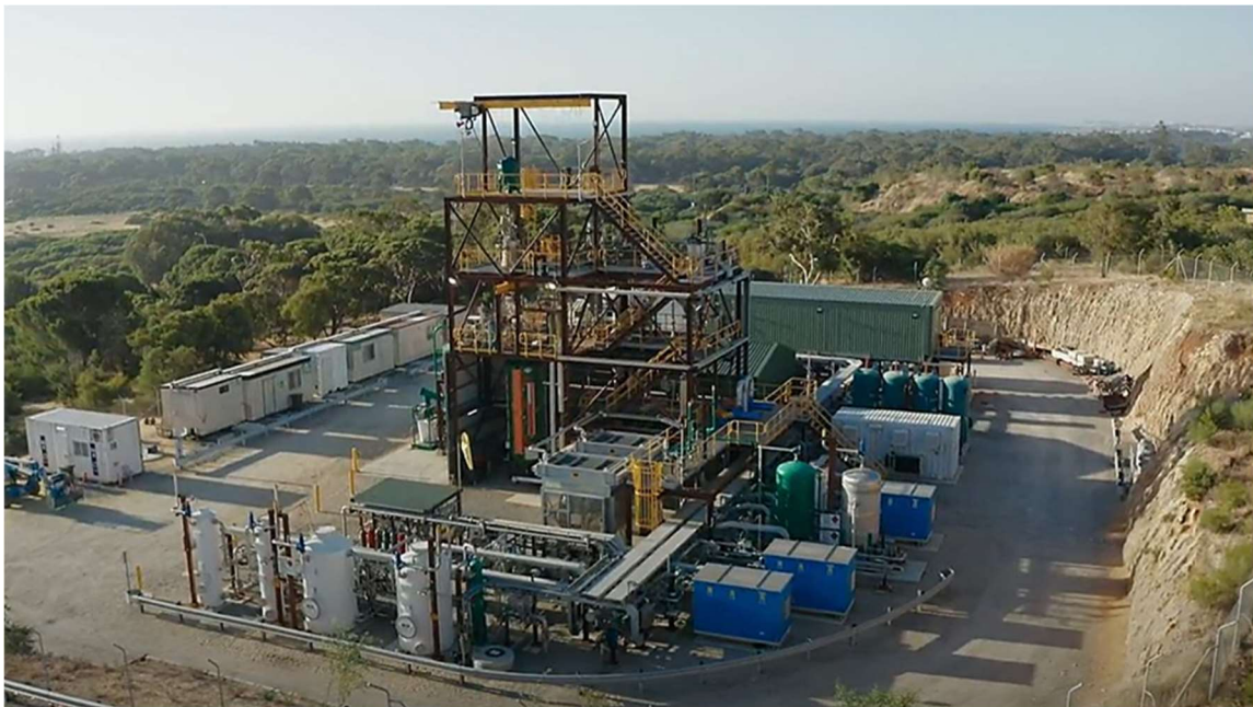
World's first commercial-level demonstration of Hazer methane pyrolysis technology producing clean hydrogen and graphite
