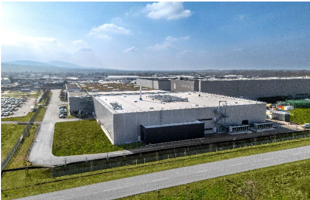
Figure 4 – Mercedes-Benz LiB Recycling Building, Kuppenheim Germany.
