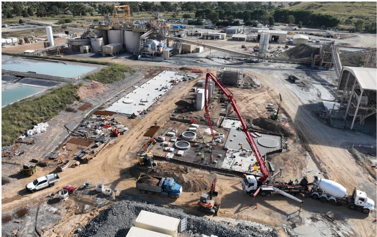
Process flotation and fine grind circuit concrete works
