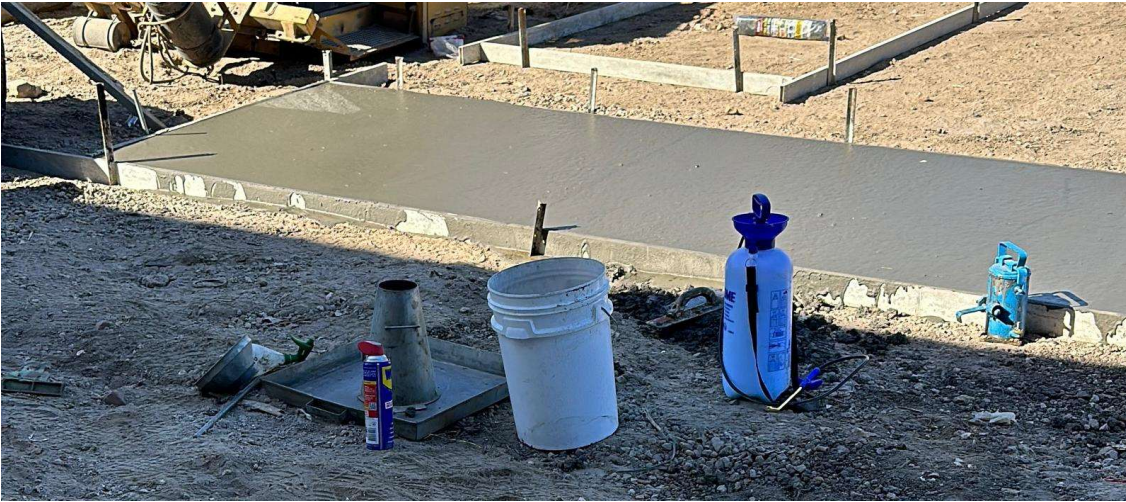
Photo 3: Prior to stripping formwork
