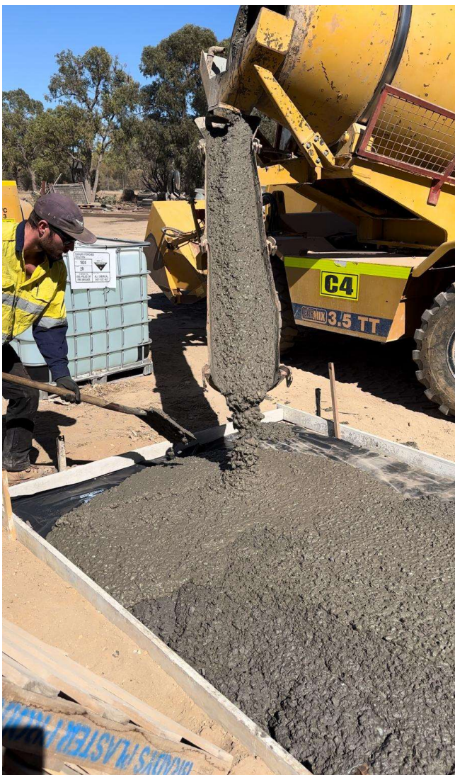
Photo 1: Pouring of Collicrete
