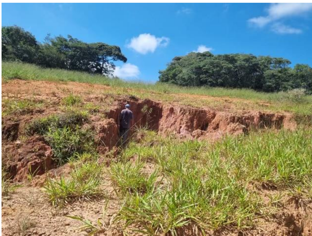
Deeply weathered saprolite clay system at T1-T2
