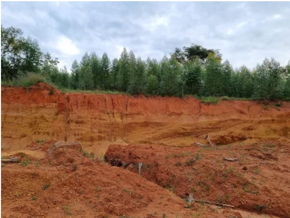
Deeply weathered saprolite clay system at T1-T2
