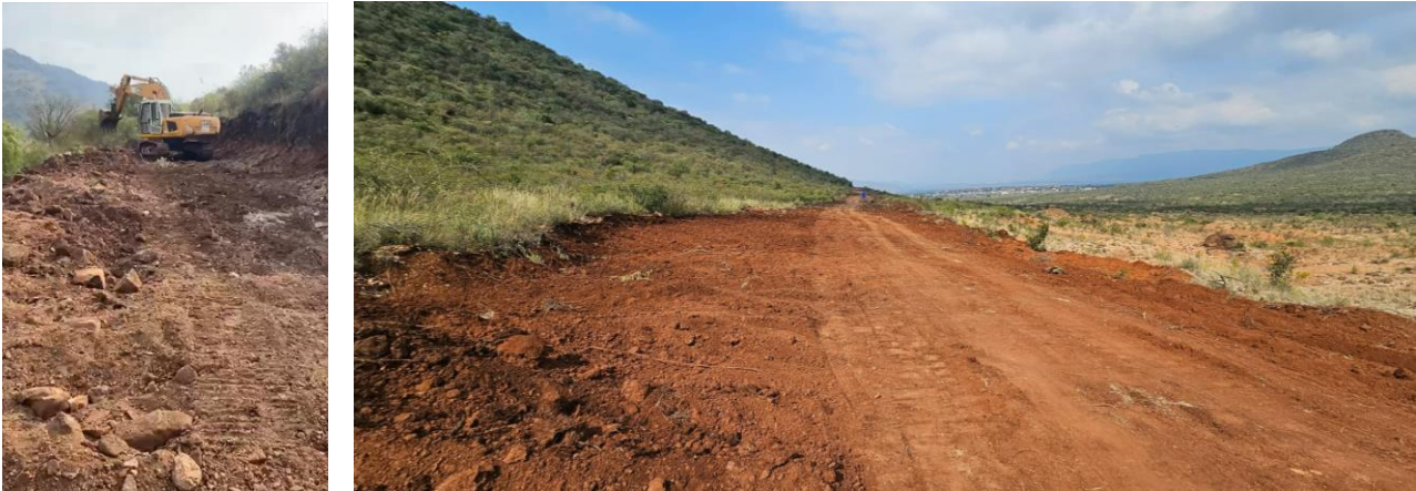
Figure 4: Site preparation for installation of boundary fence
