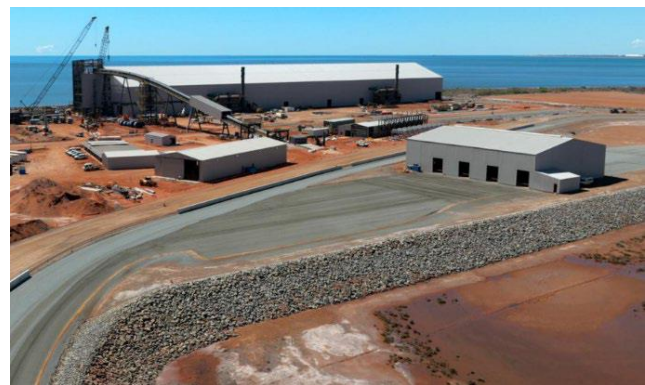
Product storage facilities at Port of Ashburton
