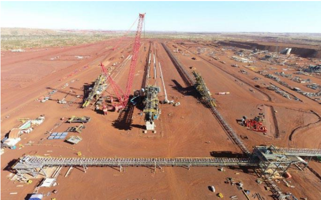
Stacker and reclaimer assembly ongoing
