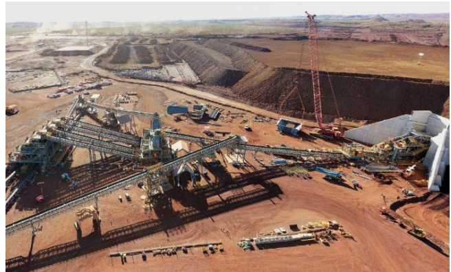
Ken's Bore crushing plant Train 3
