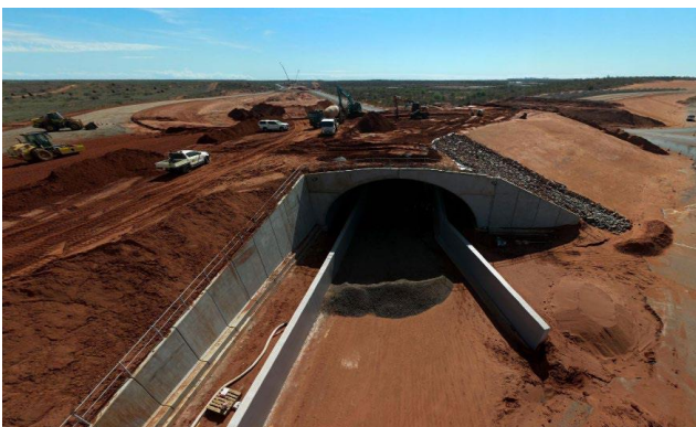
Haul road at Warrirda/Onslow Rd overpass
