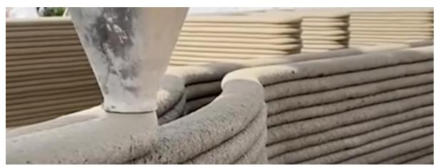
Figure 3. 3D concrete printing trial
