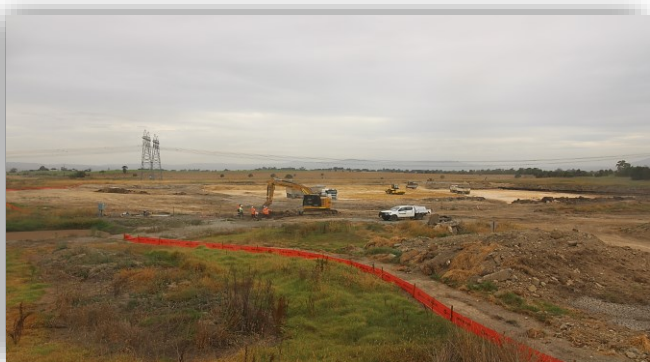
Image 3 & 4: Yarra Valley Water site works
