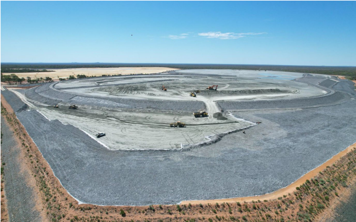
Figure 2 - CSA Copper Mine Covering Geofabric on Stage 9 Buttress
