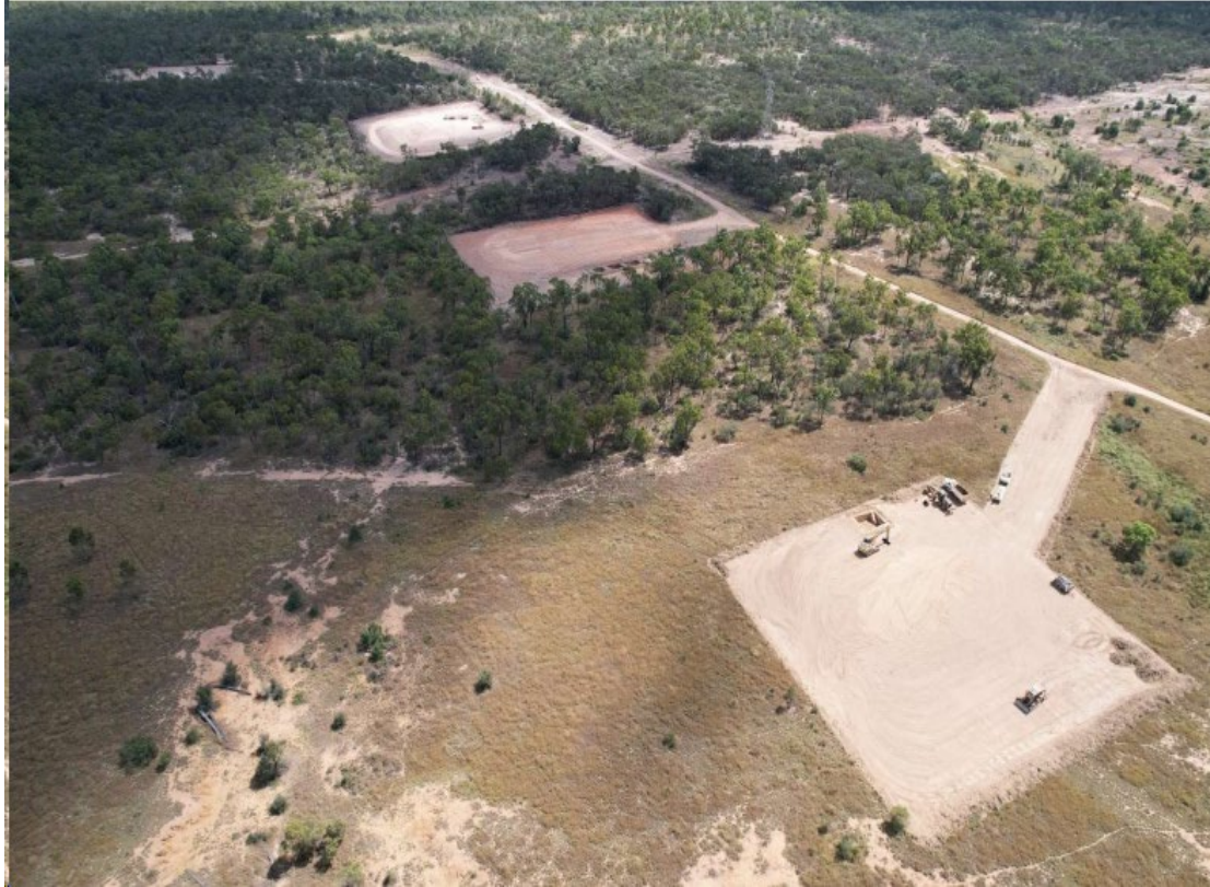
1 st three vertical well pads ready for drilling
