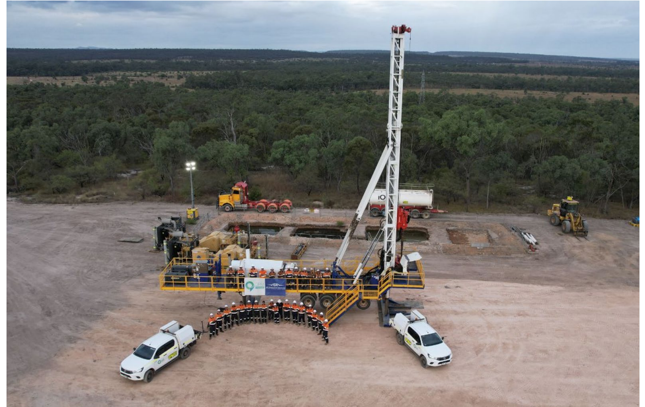
Rig – Lucas rig DRS 118 on location spudding 1 st vertical well on TB118V1
