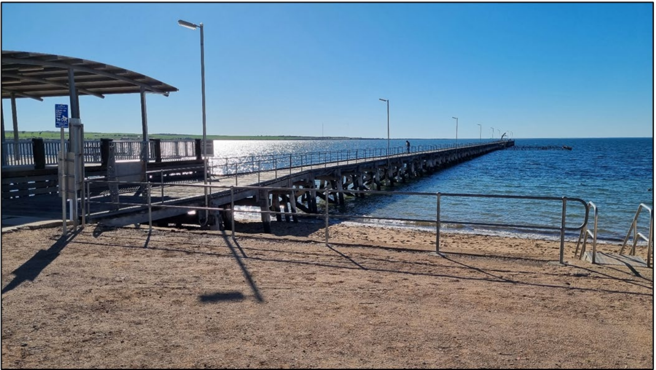
Figure 3: Trial infrastructure at Streaky Bay Jetty, Eyre Peninsula, SA
