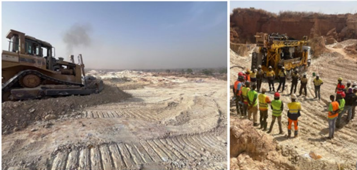
Image 2: Drill pad preparation and contractor safety briefing at the Kobada Gold Project
