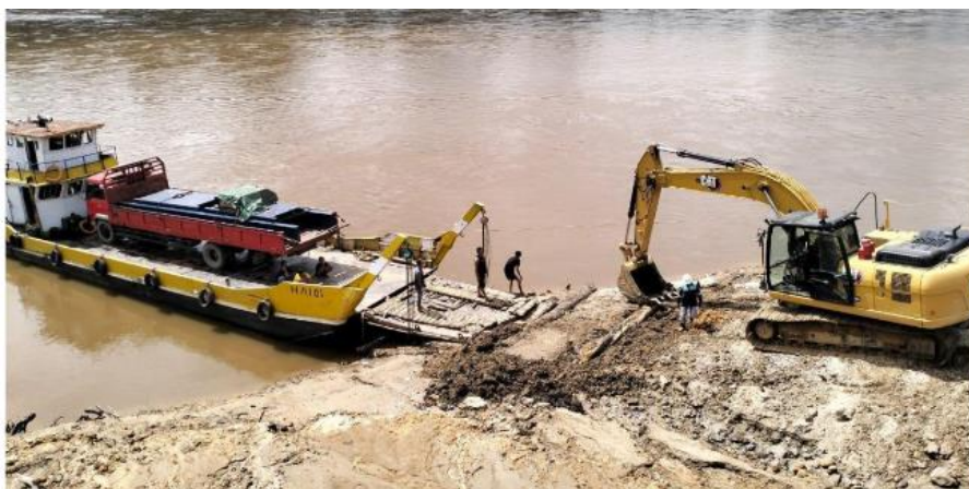
Weighbridge components being unloaded at Batu Tuhup Jetty
