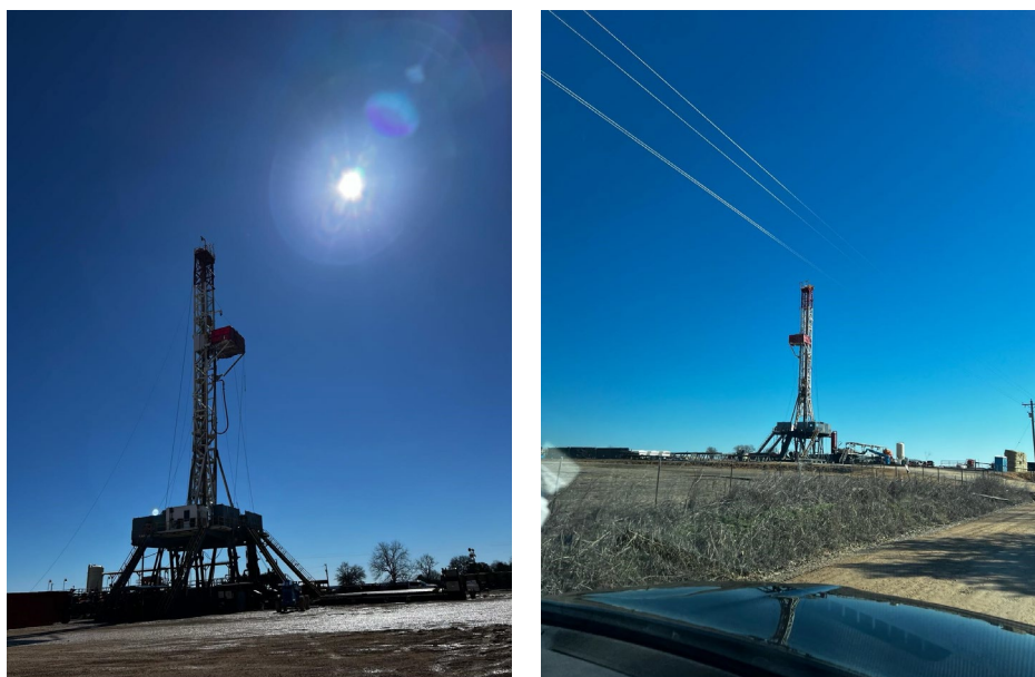
Figure 7: Kenai Rig 19 drilling the Iginla Well, Sanford Pad, Oklahoma.
