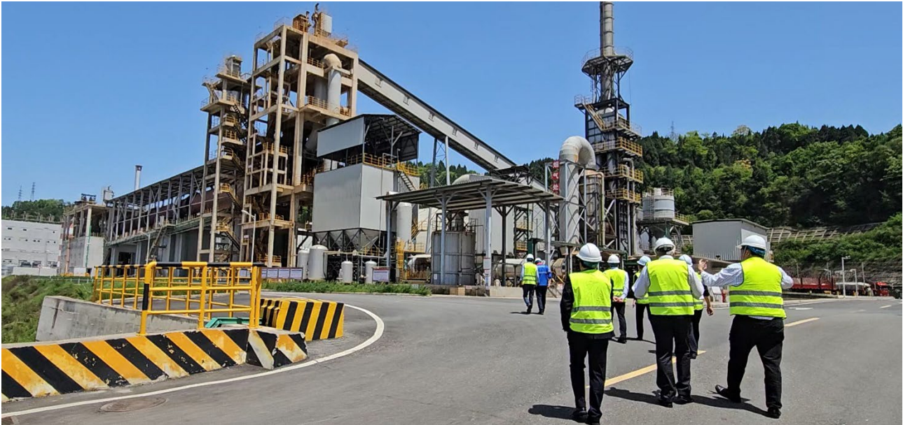
Figure 1: The Company inspects an operational lithium refinery within the Sichuan province, China.
