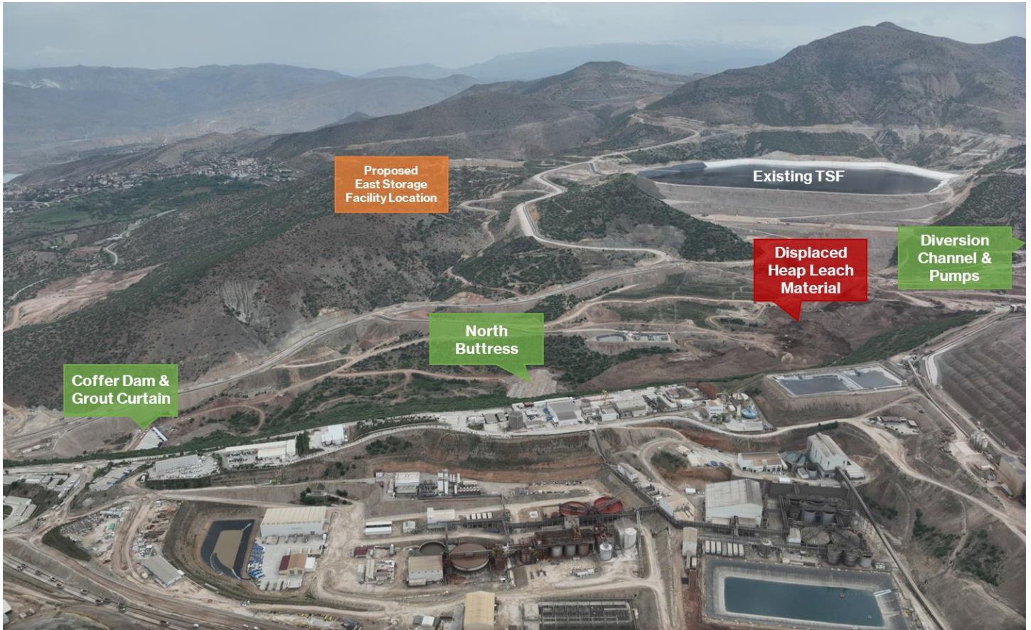
Figure 1. Location of containment and proposed remediation infrastructure overlain on an aerial view of the Çöpler site as of May 1, 2024.
