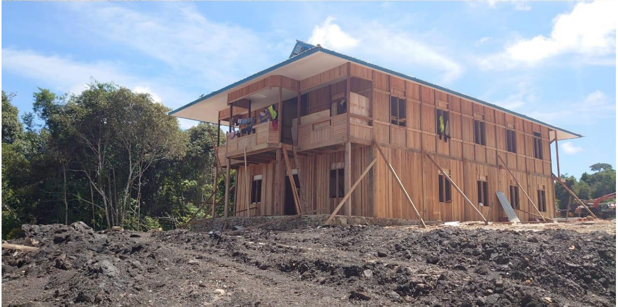
New workers camp at Pit 3
