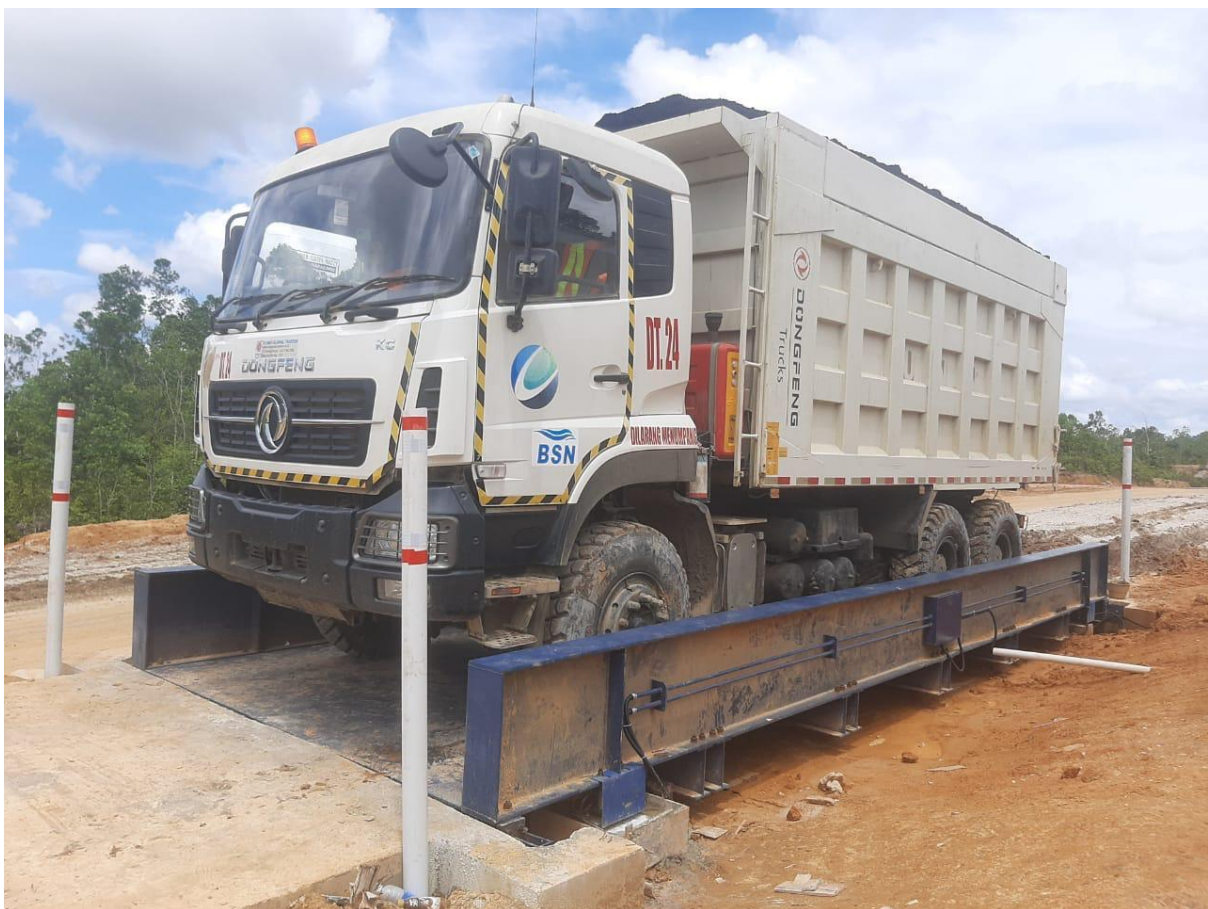
Weighbridge Batu Tuhup completed and in use.
