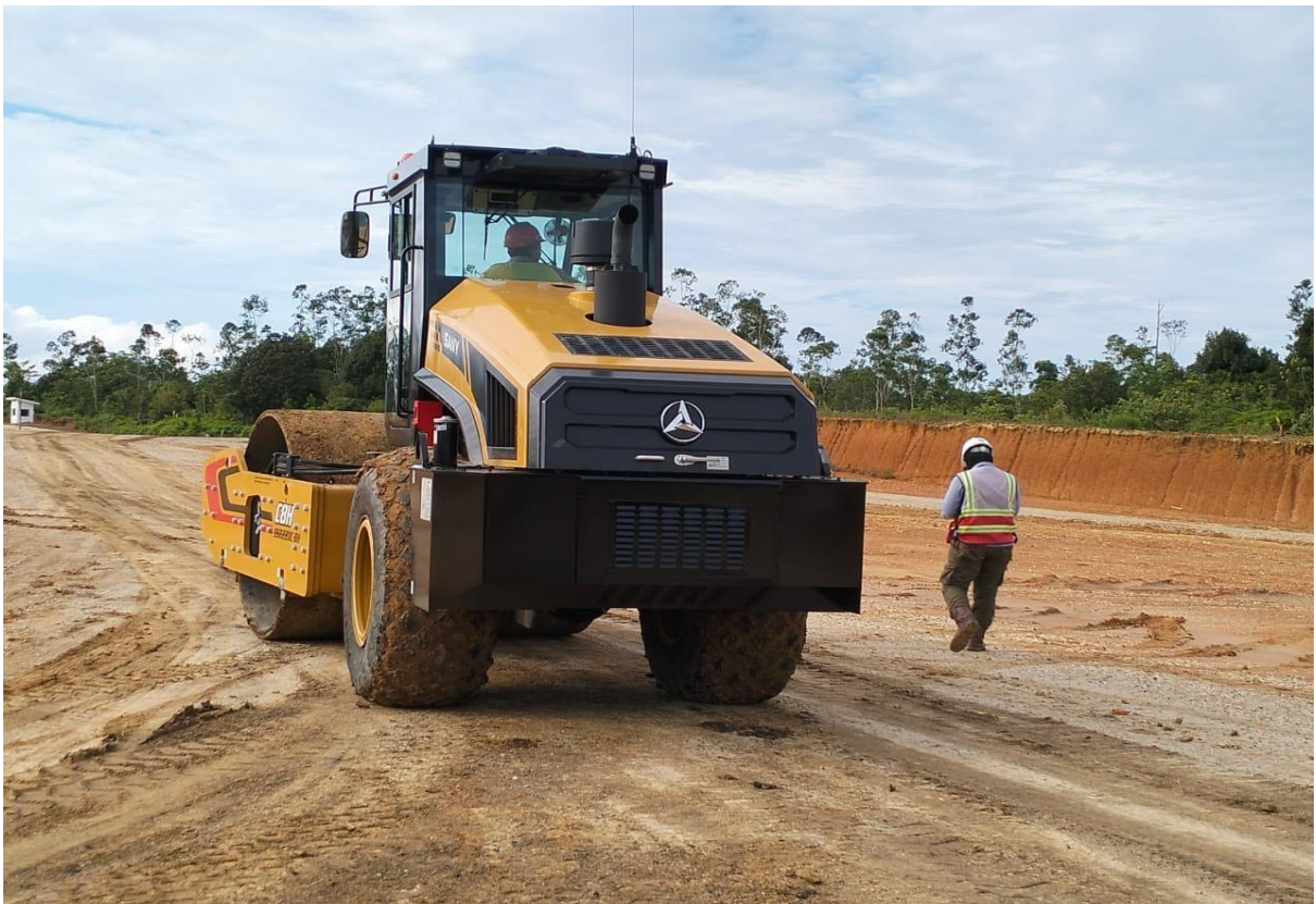
Road upgrade works at Batu Tuhup Jetty.
