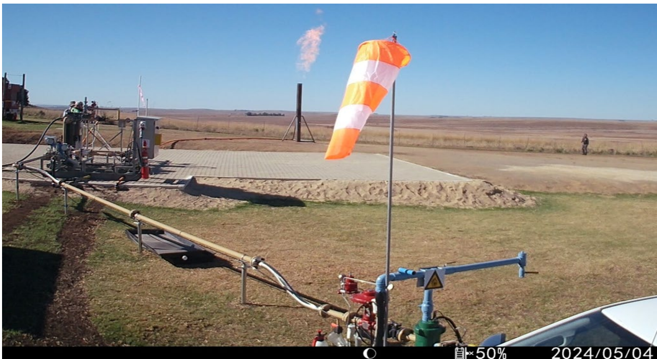
Figure 2: Well testing ahead of flow to gas generator
