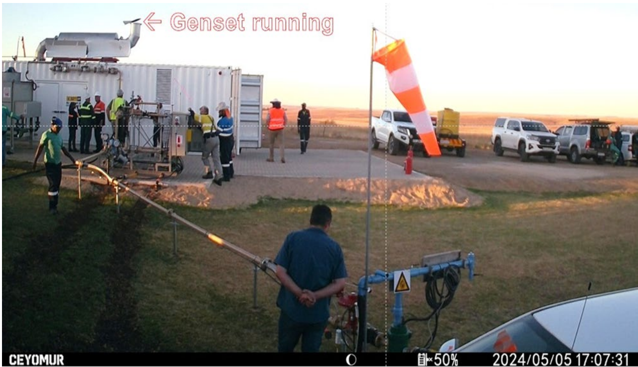
Figure 1: Gas generator powering on KKO gas flow from The Beast well
