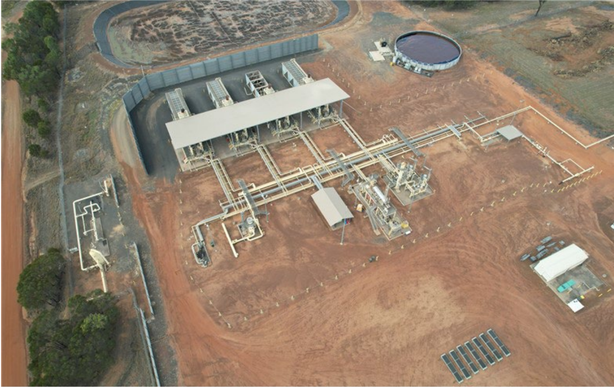
Moranbah Gas Processing Facility
