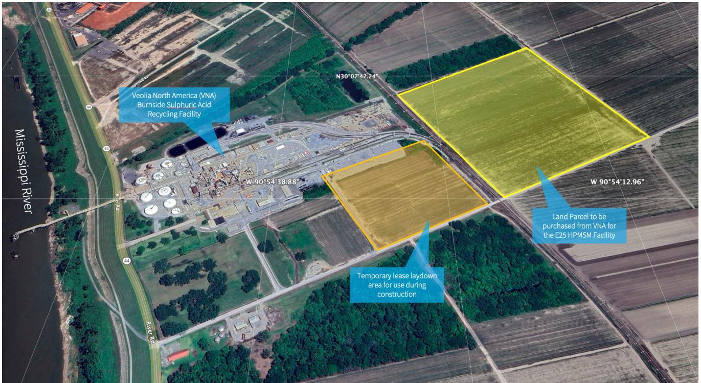
Figure 1. Proposed construction site for the Louisiana HPMSM facility close located with the Veolia North America acid plant.
