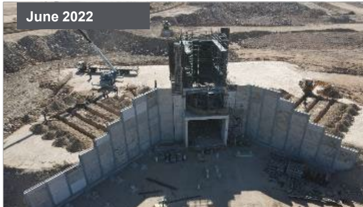
Crusher retaining wall backfill underway, ROM pad under construction
