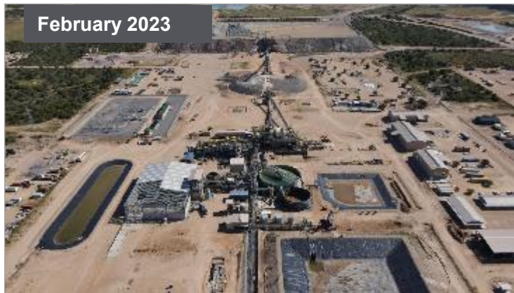
Dry plant +95% complete with commissioning activities commenced
