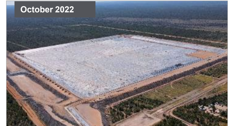
TSF Stage 1 nearing completion
