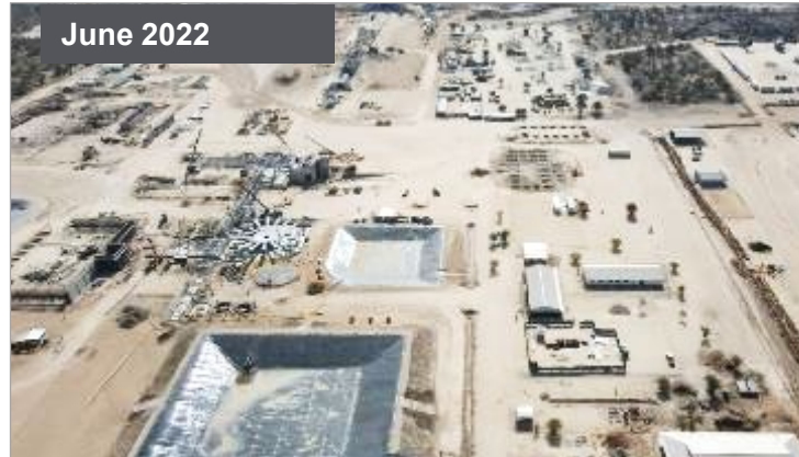
Process plant civil works 60% complete
