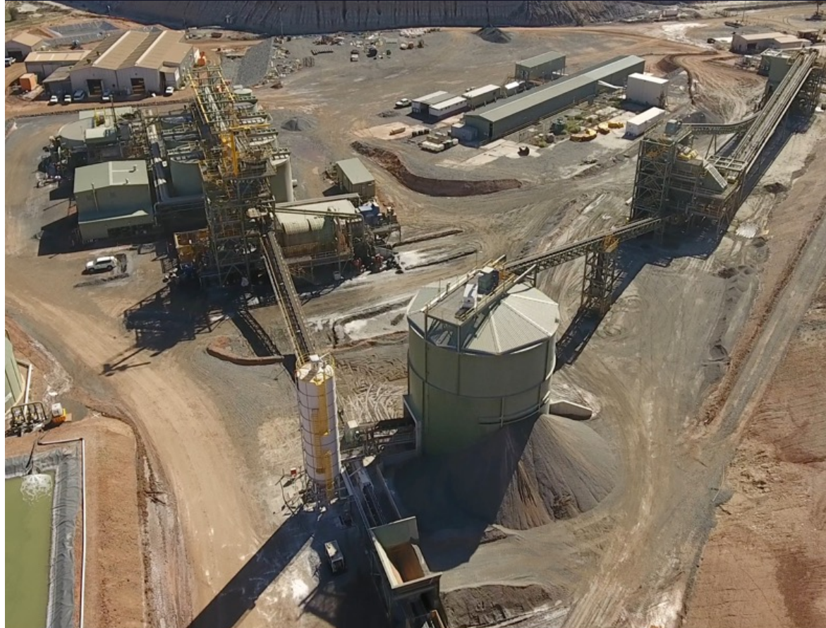
Norseman 1 MTPA processing plant is immediately expandable
