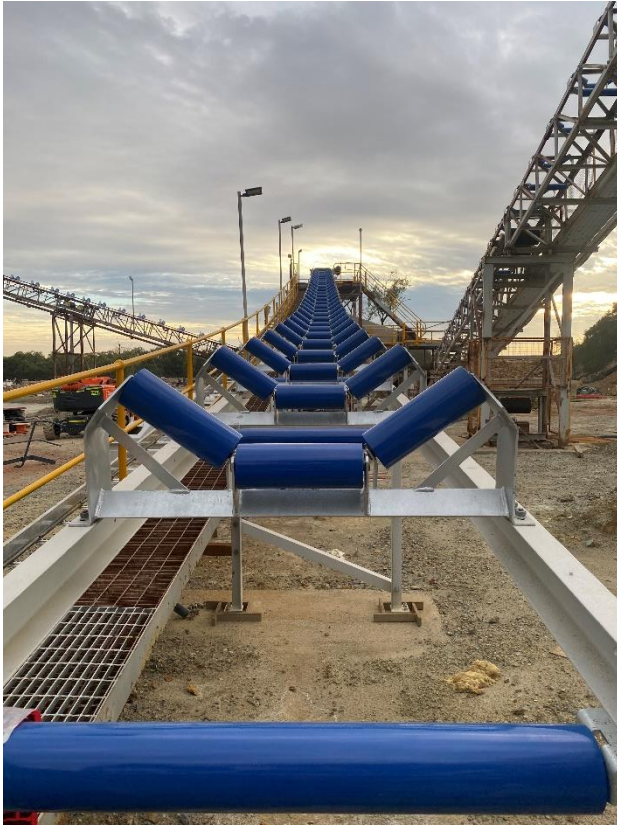
Figure 7: Mineral Hill Plant refurbishment includes – crushers & ROM bin, conveyors, fine ore bins & feeder tunnels, mills & grinding circuit, flotation plant, electrical network and supply, water supply, reagent dosing, safety equipment, instrumentation, pumps and piping.
