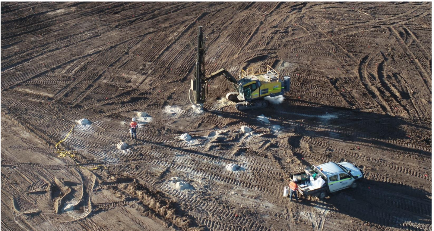
Figure 2: Pearse North open pit drilling is underway.
