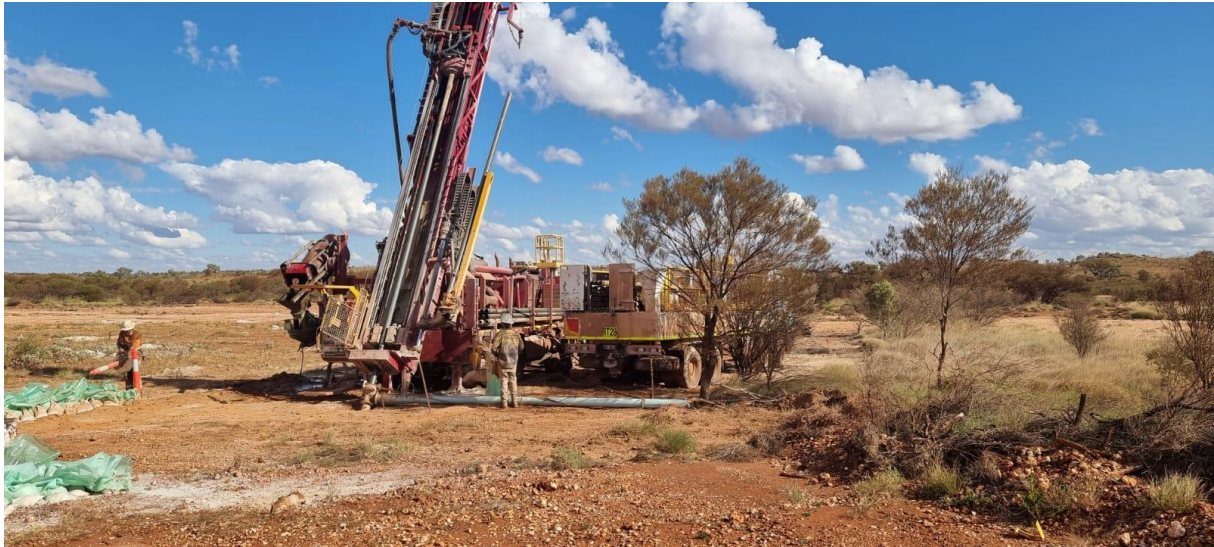
Figure 1: RC Drill Rig On Site at Tin Can Prospect (16 May 2024)
