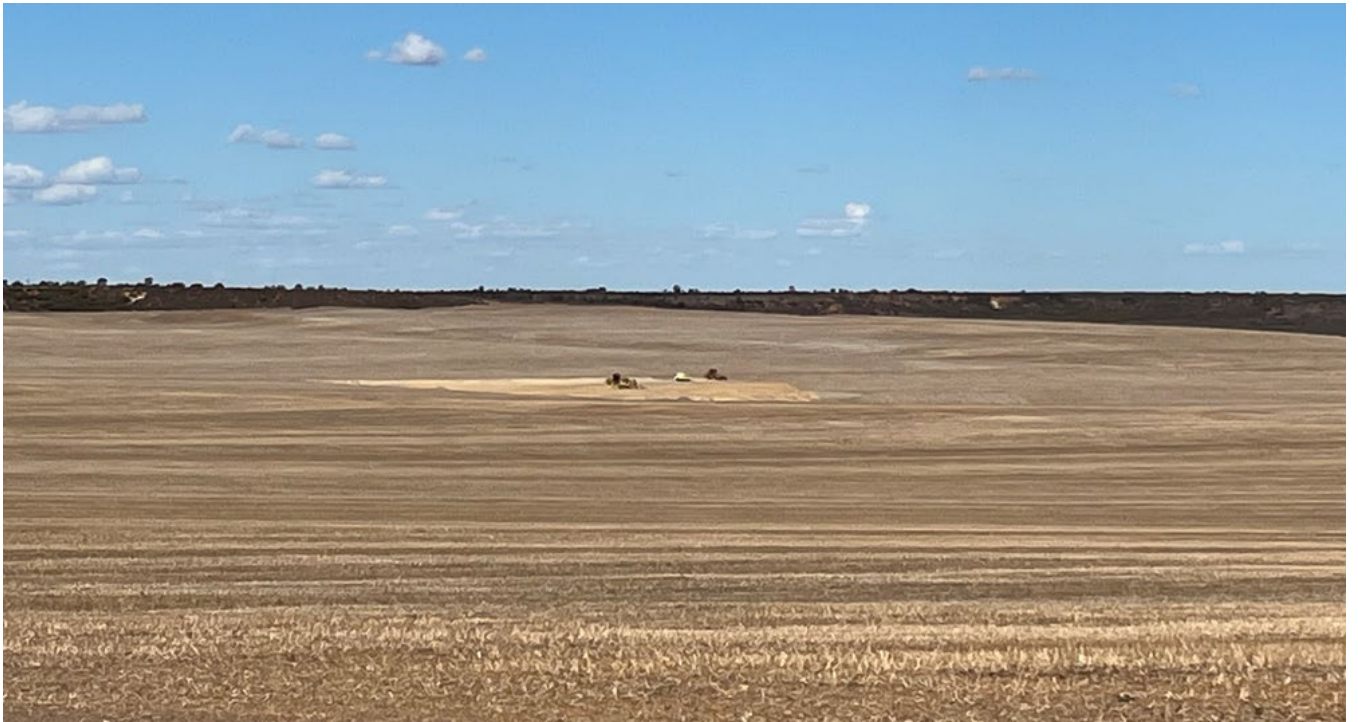
Figure 1 Booth Well Pad nearing completion
