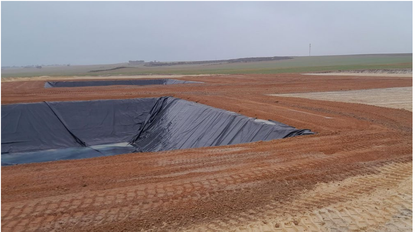
Figure 3 Booth Well Pad showing water and mud pits with waterproof lining
