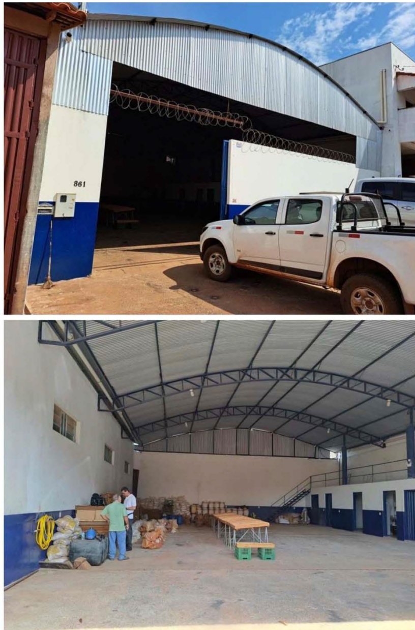
Figure 11-1 – Drill core storage shed
