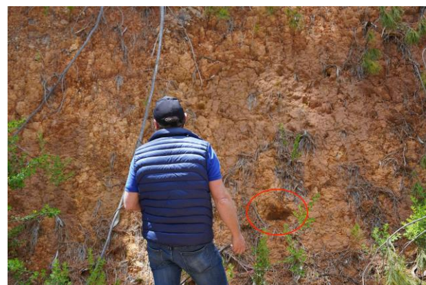
Photo 4 – Exposed clay zone with soil sample site circled red
