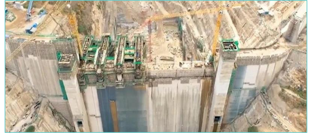
2GW Julius Nyerere Hydropower Station under construction
