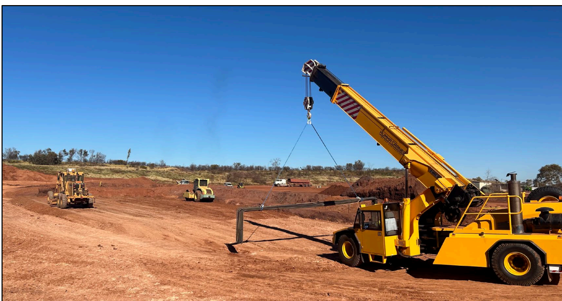
Photo 1: Construction of Nobles CIL Gold Processing Facility in progress
