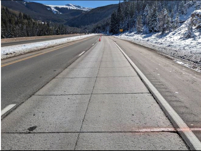
Concrete Sample Area 1, Beginning
