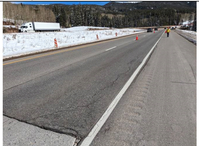
Concrete Test Section 3 to Asphalt Transition
