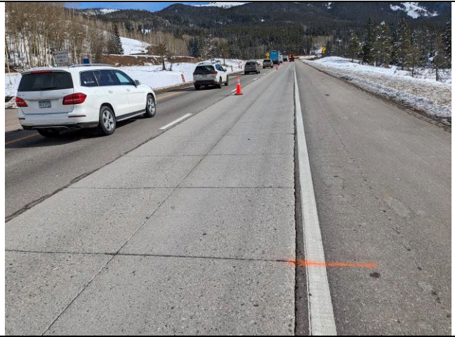
Concrete Sample Area 3 End
