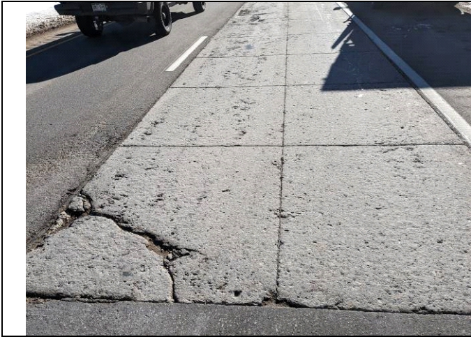
Concrete Test Section 1, First 100 Feet
