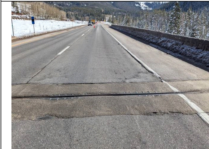
Bridge joint, F-11-AM
