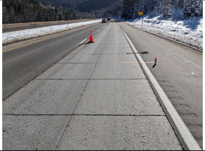
Concrete Sample Area 1, End
