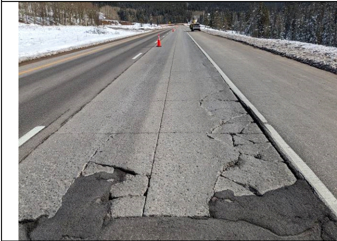
Concrete Test Section 2, First 100 Feet
