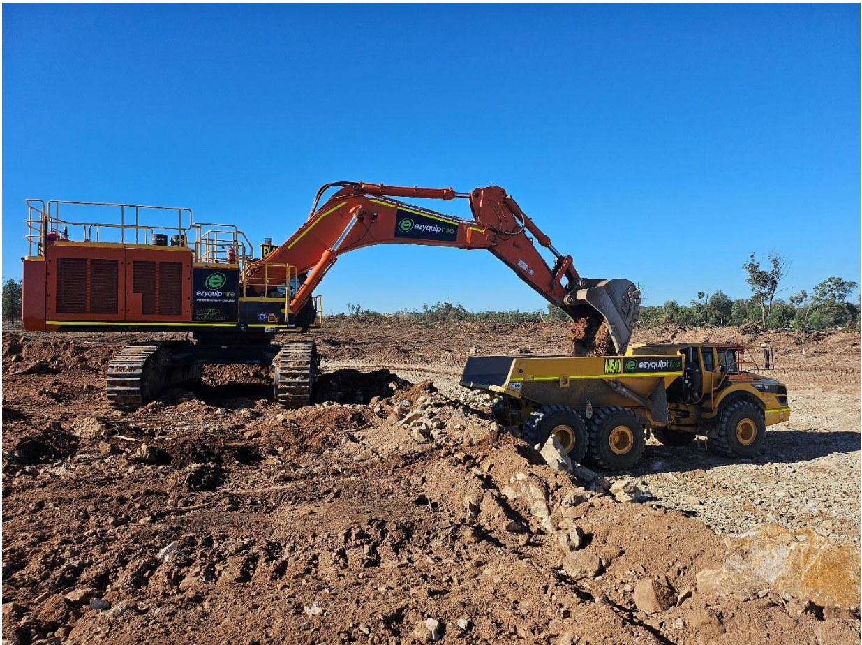
Figure 4: Open pit excavation and haulage.
