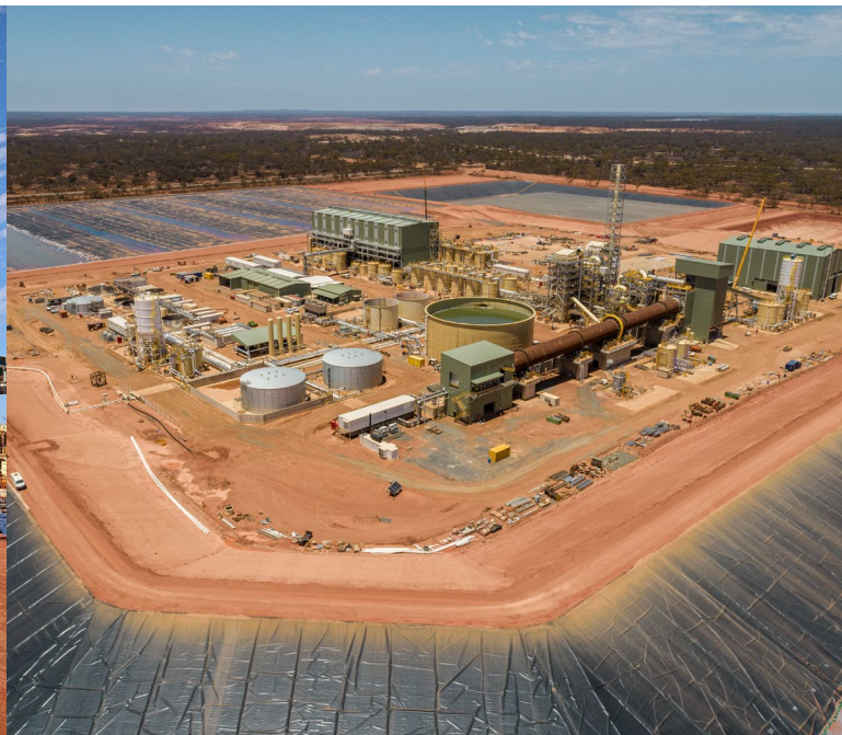
New Kalgoorlie Rare Earths Processing Facility
