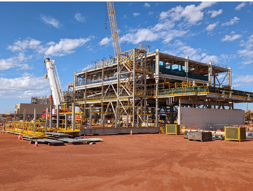
Mt Weld Expansion
