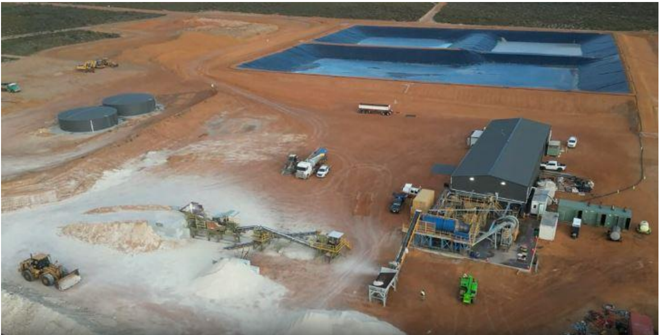
Figure 2: Kat Gap Processing Facility.
