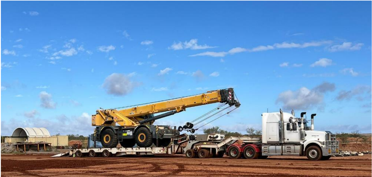
Figure 1: MACA equipment being unloaded at site, including 60t Rough Terrain crane.
