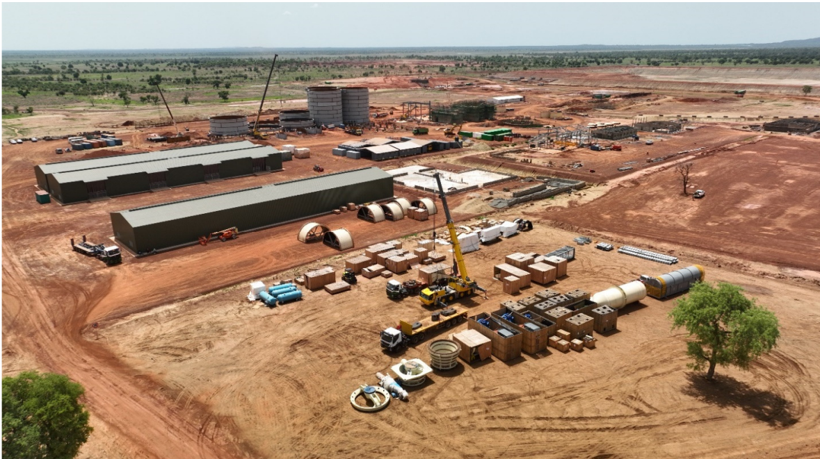
Figure 1: Construction of the process plant infrastructure at Kiaka (June 2024)
