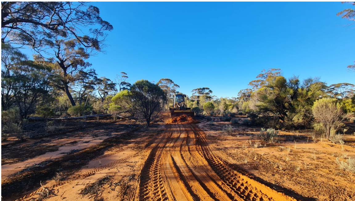
Figure 1. Loader clearing new track to drill pad at the Koolyanobbing Fe Project
