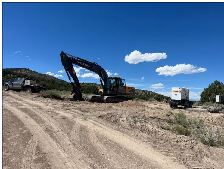
Figure 1 - Laydown area construction and Water Bore installation
