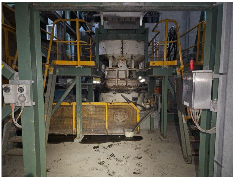
Figure 4: Terex cone crusher and local infrastructure
