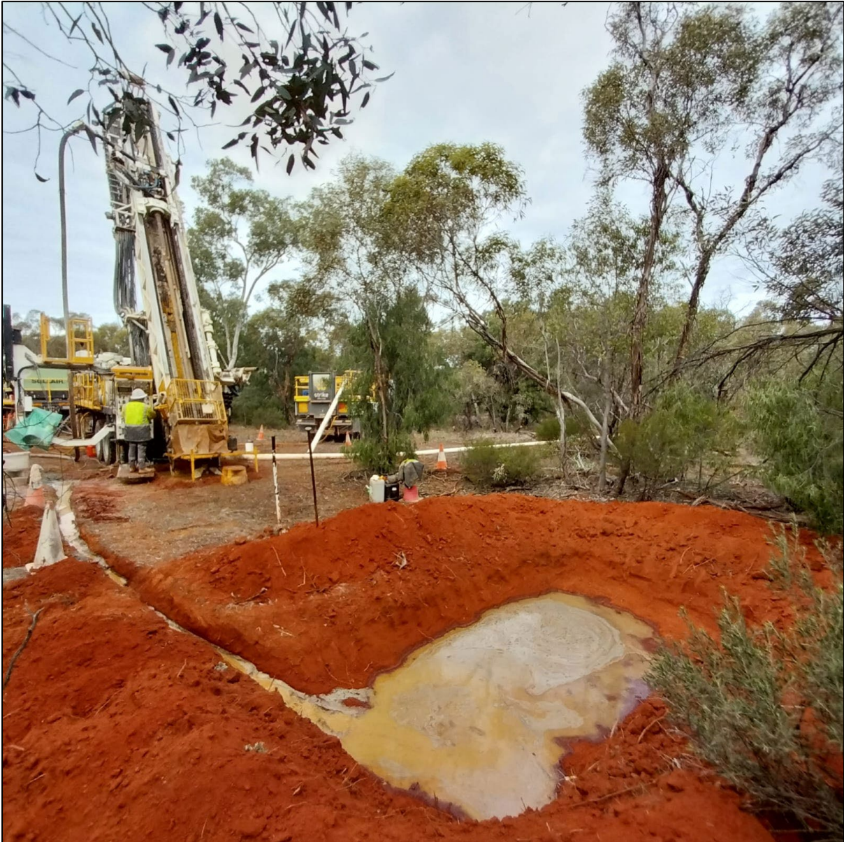
Figure 2: Photo of drill rig at hole A3RC044 showing water management controls in the foreground.
